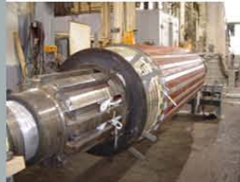
Generator evaluation being performed at our extensive Columbus, Ohio facility.
